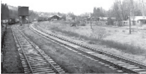
Union Pacific railroad track at Gibbon (26.5 miles from Kamela (west of La Grande), 1940s Photo courtesy of John Turner and Richard Hermens
